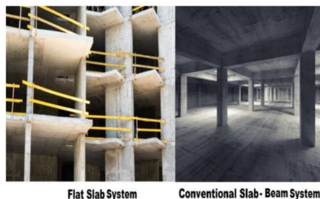
Fig: Shows the flat slab system and conventional slab-beam system
