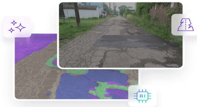
Figure 4: Overview of the AI-powered analysis pipeline used in our deployed system.
